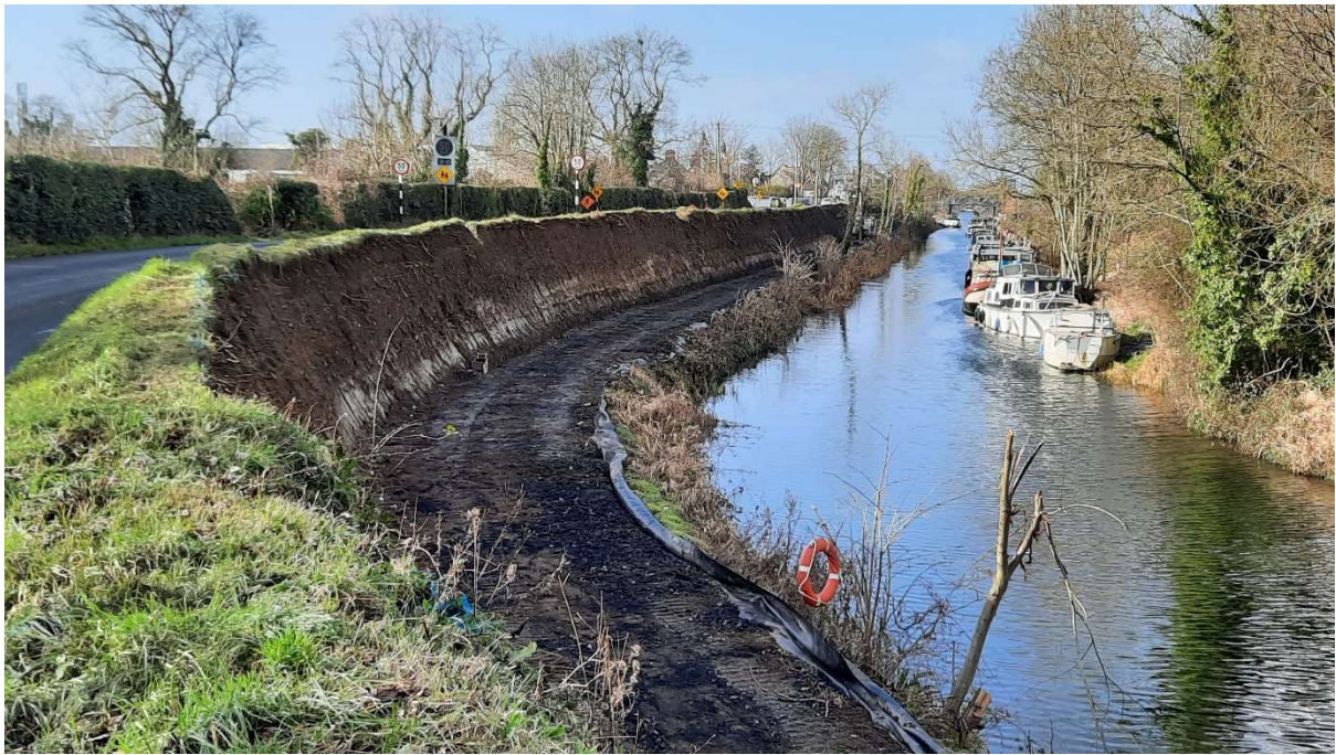
At Sallins - Work ahead of the soil nail installation
