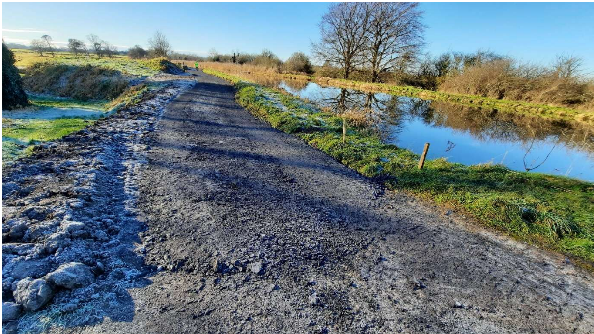
Sallins Railway Bridge to Devonshire Bridge Section
