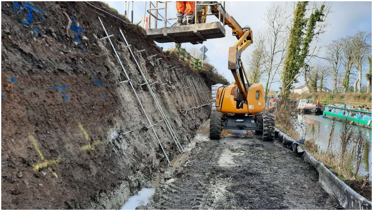
Soil Nailing Reinforcement Works at Sallins
